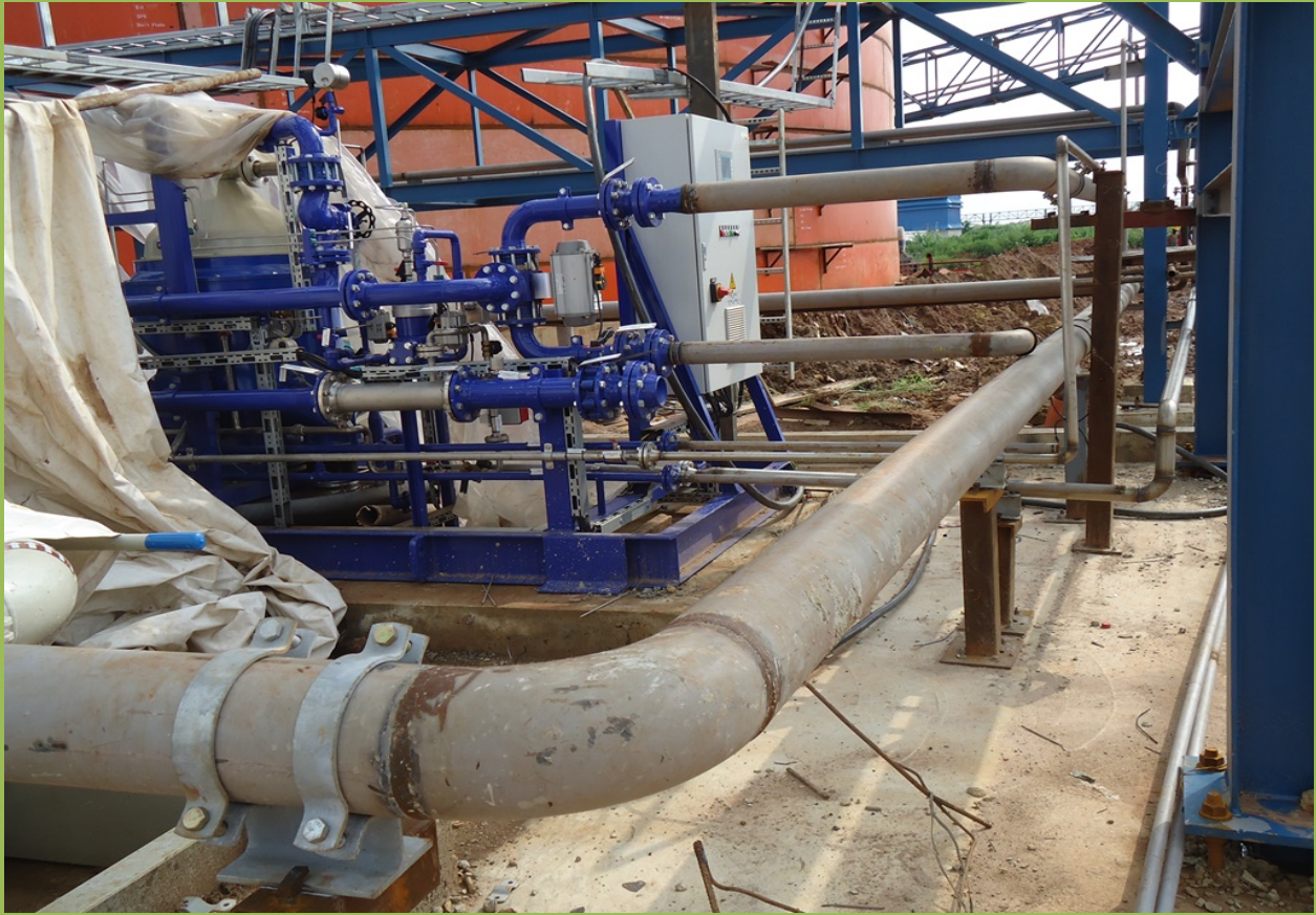
Diesel Recirculation Unit Installation & Piping
