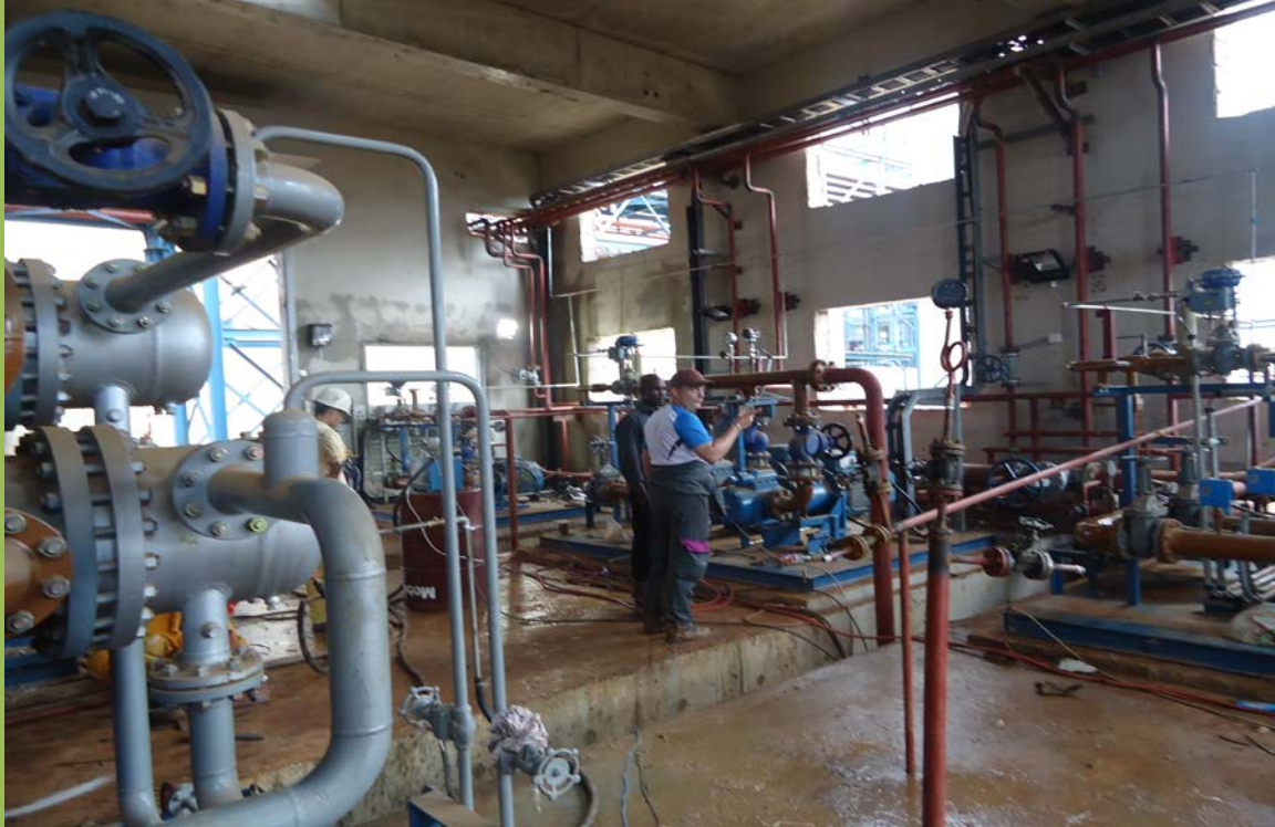
Fuel treatment house under construction for Dangote Cement Plant, Ibeso
