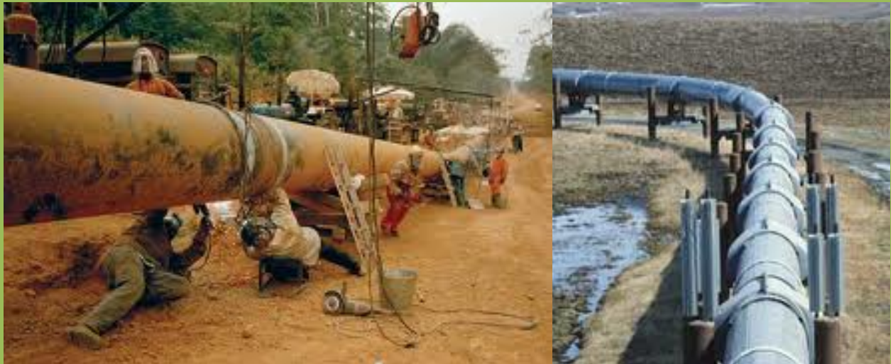
Onshore pipeline under Construction for Agip at Samabri/Biseni cluster location
