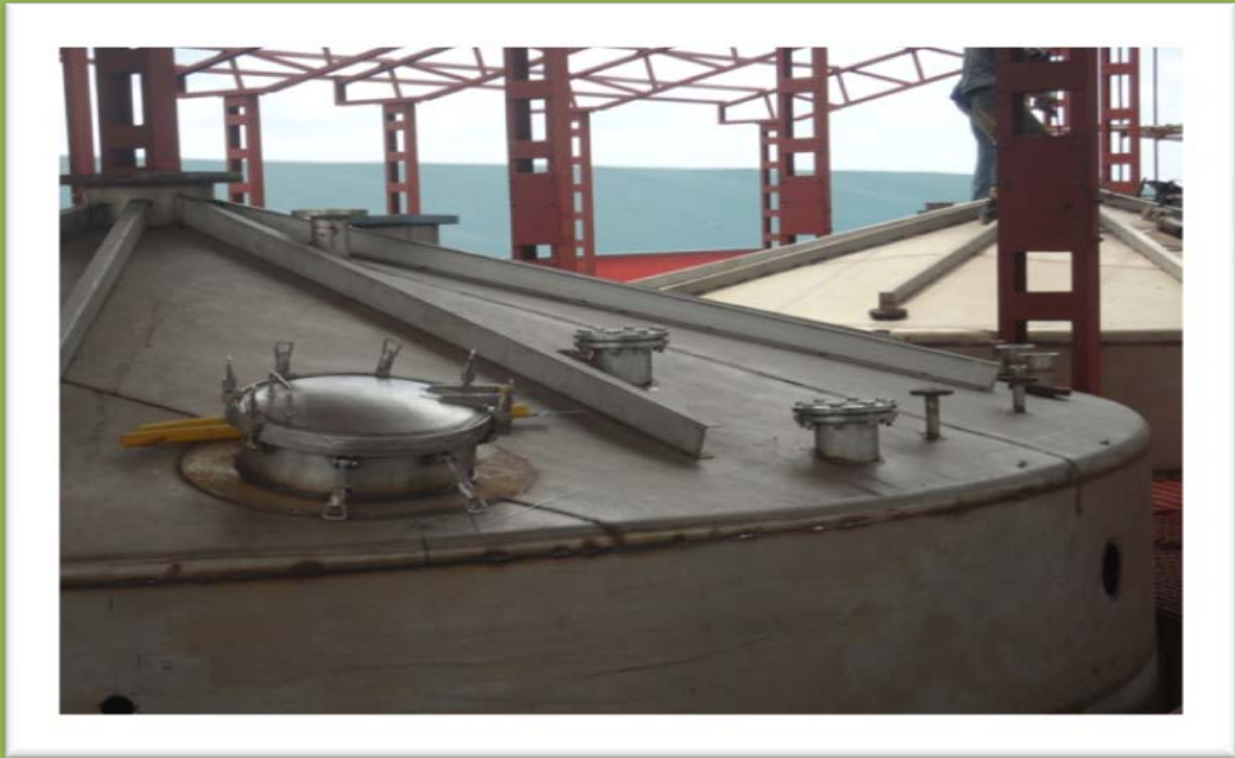
Fermentation Tank Fabrication & Installation For Nigeria Brewery Iganmu plant.
